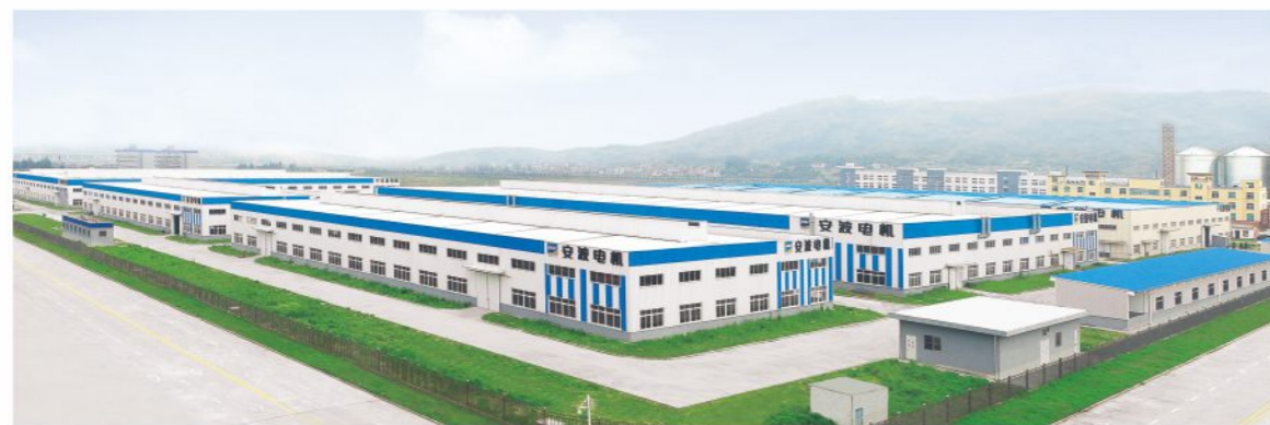
▪ 宁德工厂 Ningde Factory
