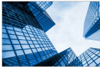
楼宇供水 Building water supply
